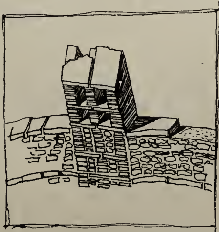
FIG. 60. Ribs in the cupola of the so-called Temple of Minerva Medica at Rome.
